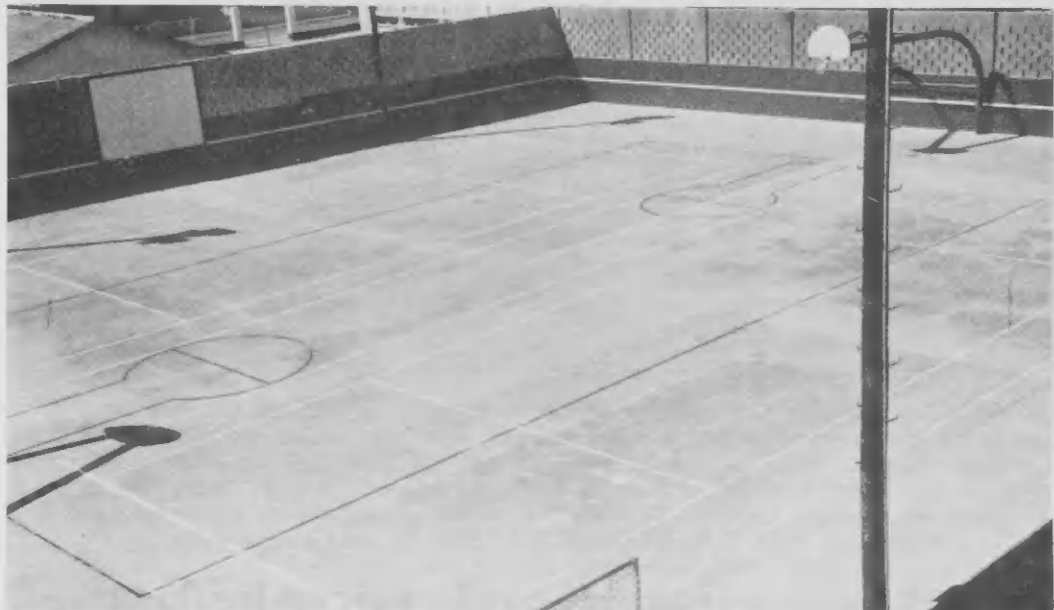
THE ENTIRE court area of the Lago Sport Park facilities was renewed with a five and one-half-inch layer of concrete. The huge pour was completed at the end of the year, which allowed time to organize the island-wide volleyball tournament as the first activity on the new surface. Ten girls' teams are participating in the play.
